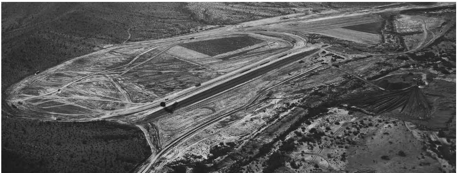
Photo credit: Getty Images, Racetrack construction circa 1963.
